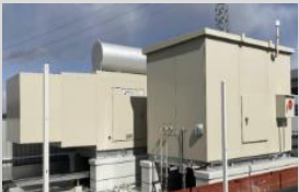
▲ Emergency in-house power generation system
